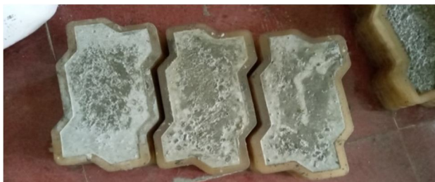
Fig 2. Casting of Paver blocks
