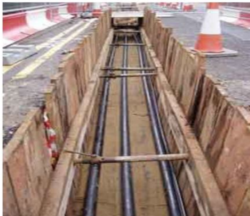
Fig 2: Underground cable laying
