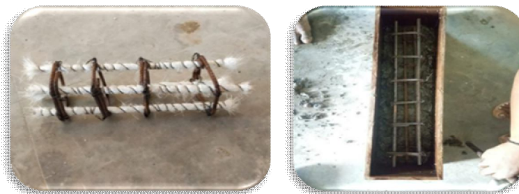
Fig 4.4 Preparation of CSGN & CSGS Concrete Column
