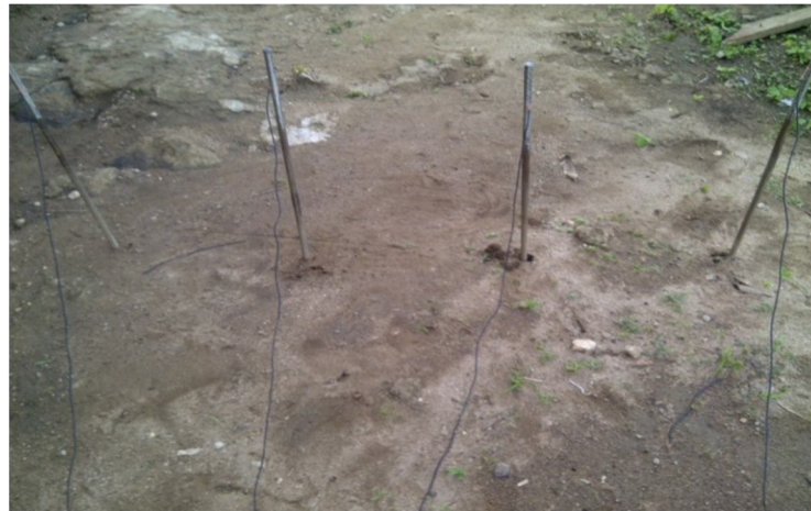
Fig. 3. Four electrodes placed in the ground
