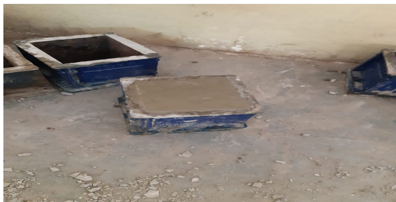
Figure: Casting of Concrete
