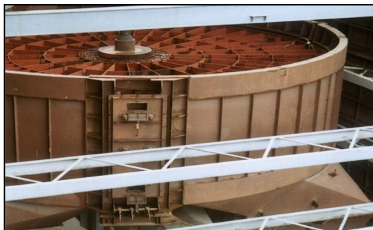
Fig.3: Thermal Wheel
