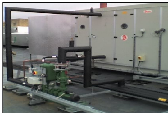
Fig.2: Run-around Coil
