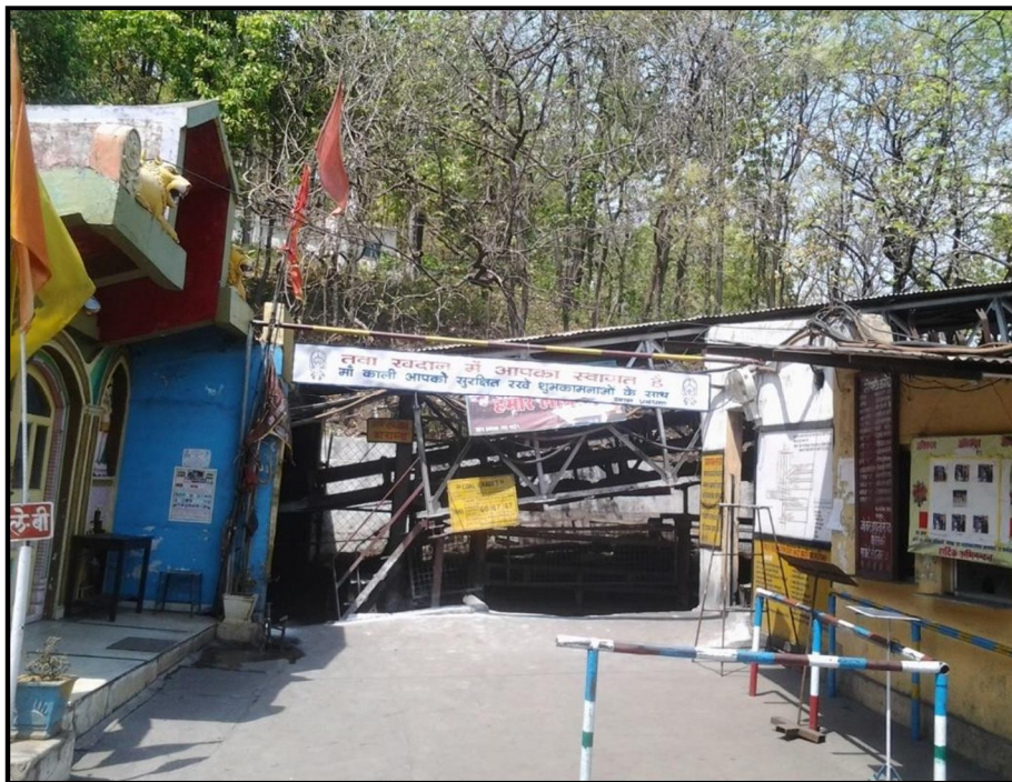
Figure 3:Tawa Coal Mines of Western Coal Fields Ltd., Betul (M.P)
