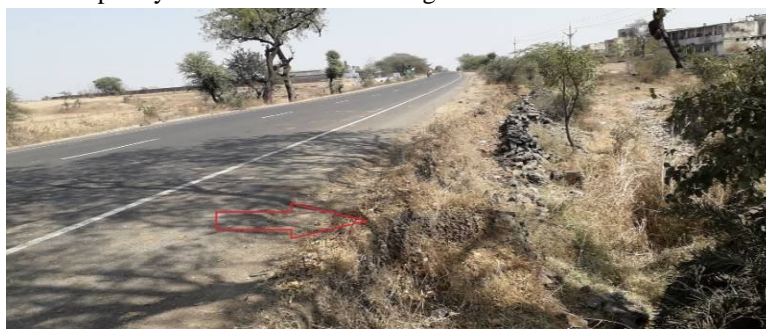
Figure 3:- steep embankments at near dondwada village.
