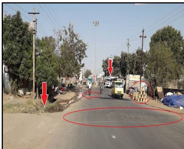
Figure 2:- Passenger boarding and alighting, Drainage problem, road side activity, non-engineered speed breaker at intersection.at bhairaw mandir square
