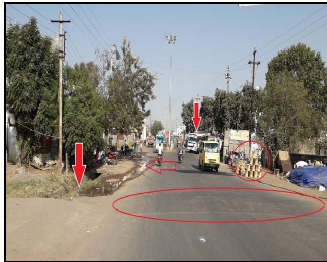
Figure 2:- Passenger boarding and alighting, Drainage problem, road side activity, non-engineered speed breaker at intersection.at bhairaw mandir square
