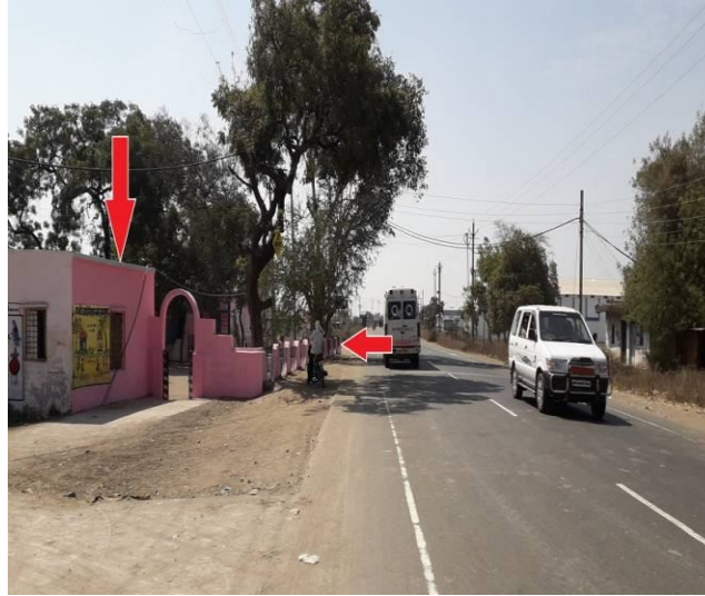
Figure 4:- School is very close to highway at Dondwada village (SH-26)
