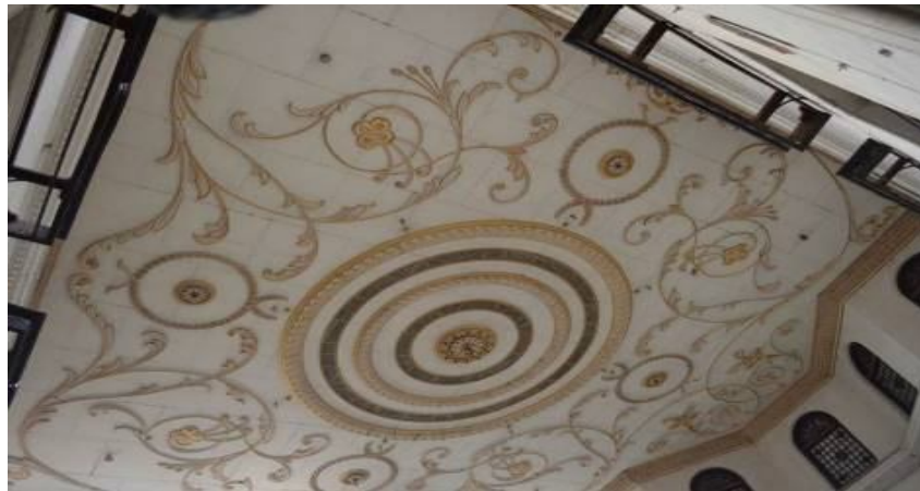
Fig. 35 The Gold Gilding work on the Ceiling
