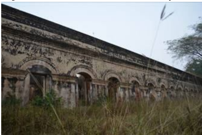
Fig. 23 Wall with Segmental Arches
