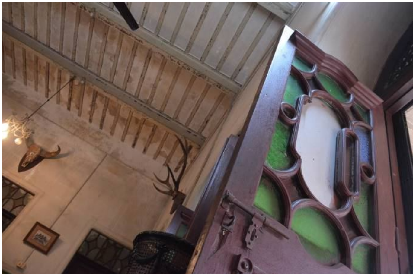
Fig. 26 Iron Girder Ceiling and Wooden Door
