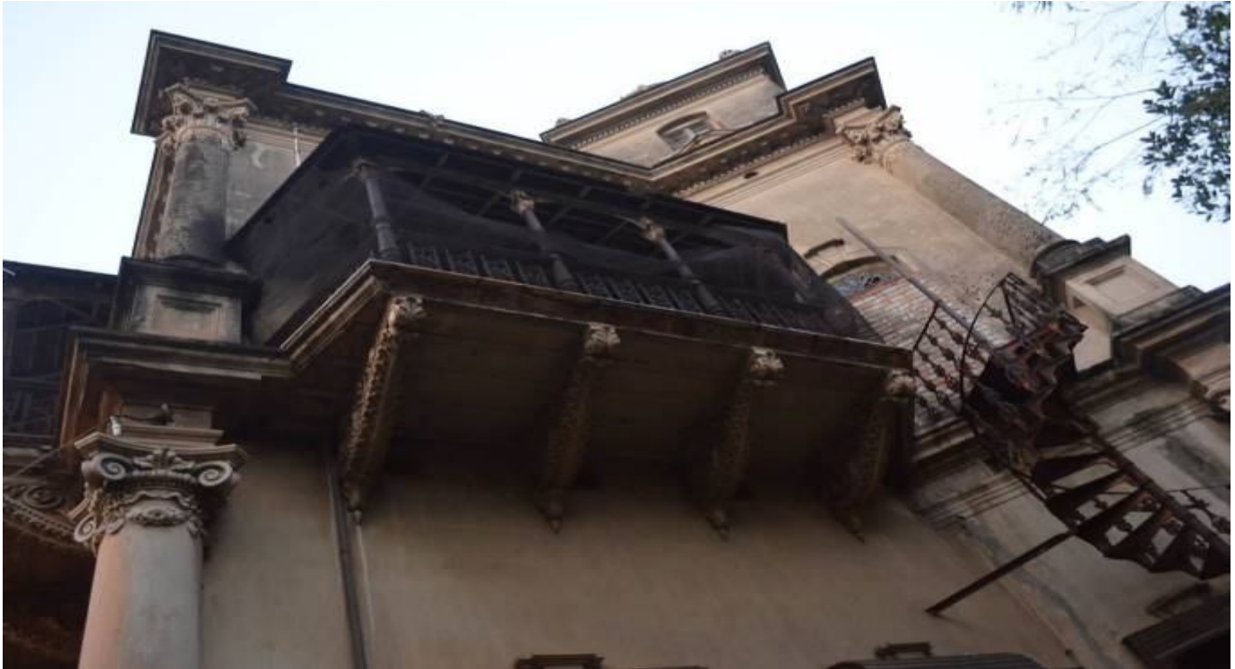
Fig. 25 Cast Iron Spiral Staircase and Balcony with Cast Iron Railing
