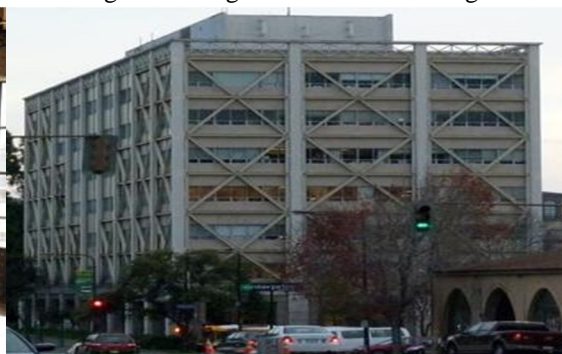
Figure 4: Showing bracing as retrofit solution
