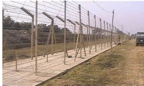
Fig. 2 Image of fencing at indo-pak border [11]
