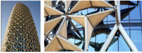
Fig.4: Al- Bahr Towers, Abu Dhabi, United Arab Emirates By; Aedas Architect
