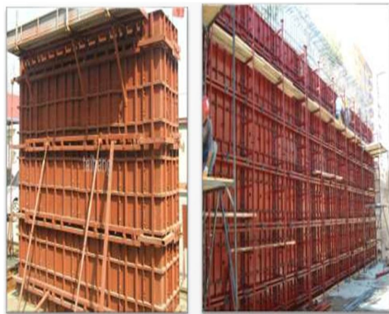
Fig. 2. Steel Formwork
