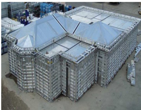
Fig. 3. MIVAN Formwork System
