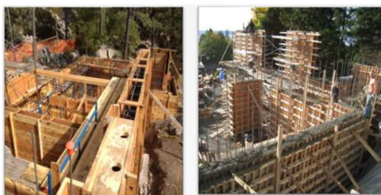
Fig. 1. Wooden Formwork
