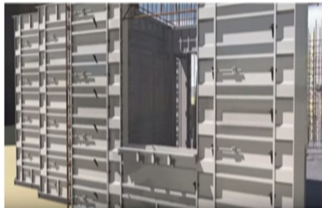
Fig. 5. Placing of formwork
