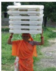
Figure 3: Worker easily carrying 6 slabs of plastic formwork
