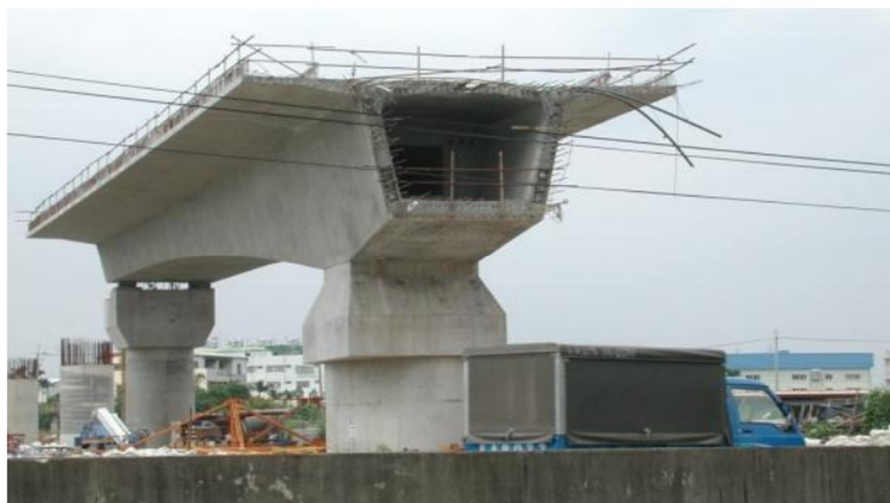
Figure 1: Box Girder Bridge
