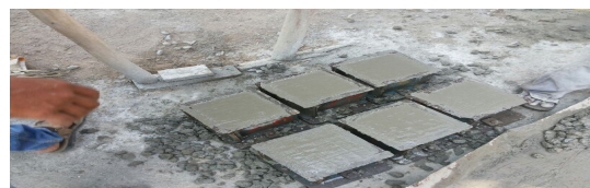
Fig-4 Casting of cubes
