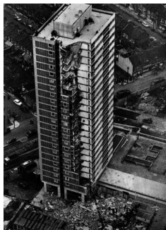
Fig 1 collapse of a part of the Ronan Point apartment
