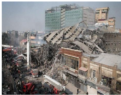
Fig 2 Plasco Building Progressive Collapse
