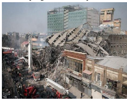
Fig 2 Plasco Building Progressive Collapse
