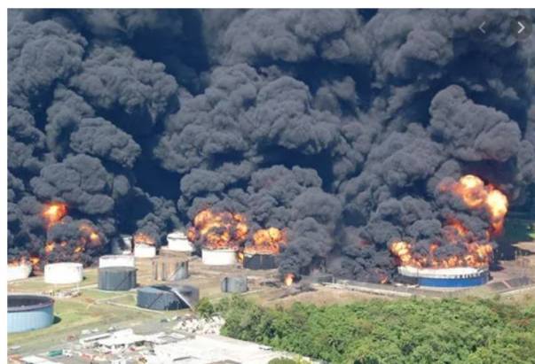
Figure 2: Industrial disaster due to gas leakage.
