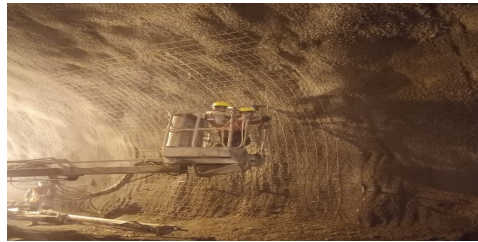
Figure. Installation of Wire mesh
