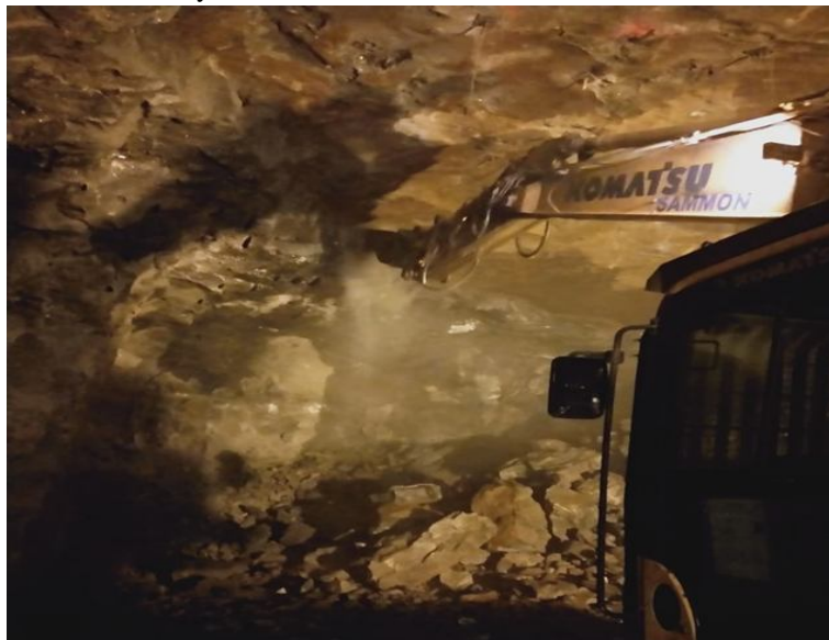
Figure Scaling & Trimming
