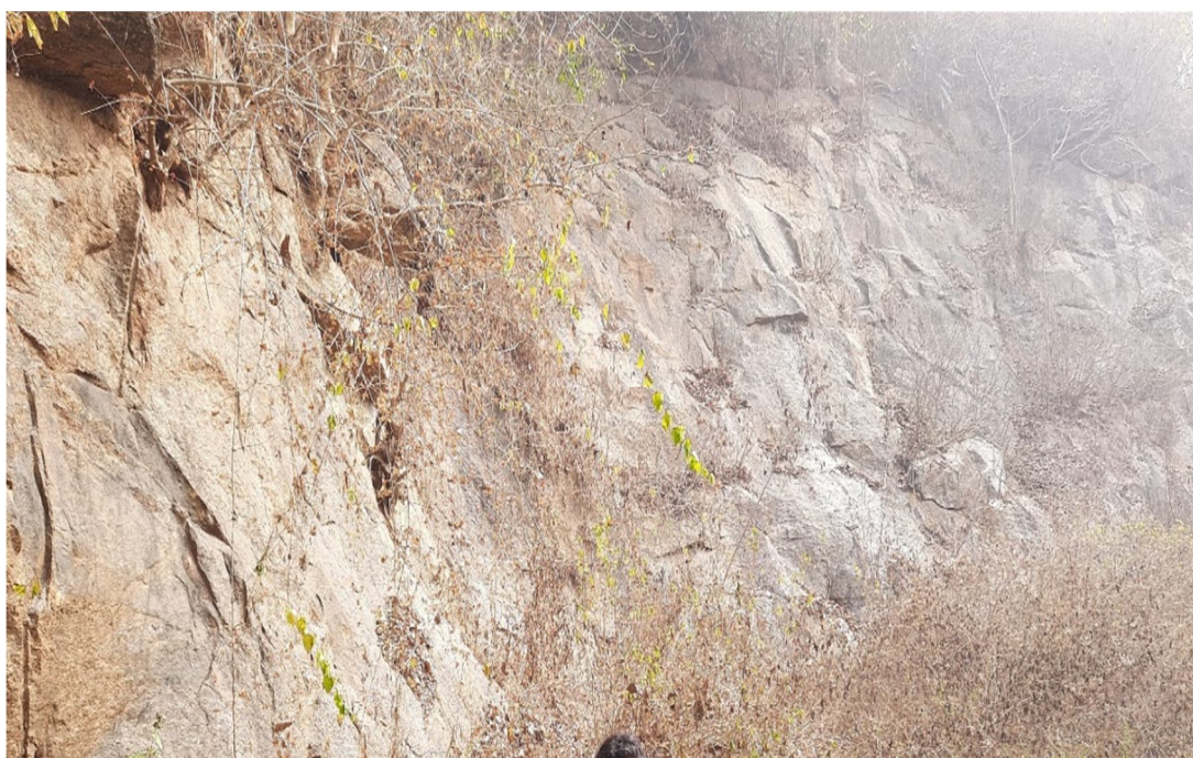
Fig. 7 Field photograph showing one set of less prominent joint in massive granite
