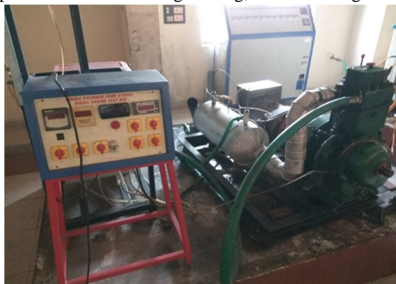
Figure no:- 4 Electric Panel
