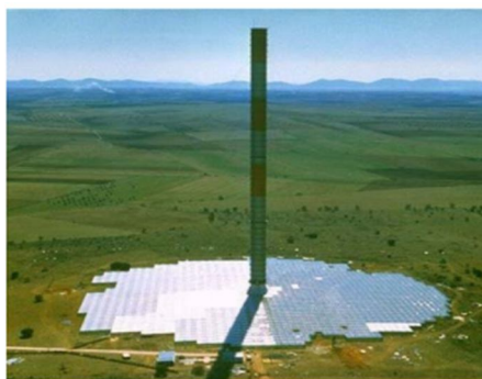
Fig 4. Prototype of the solar updraft tower at Manzanares, Spain [2]
