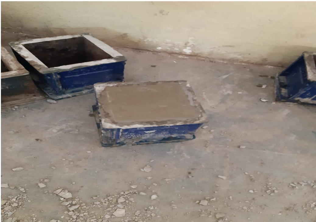
Figure: Casting of Concrete
