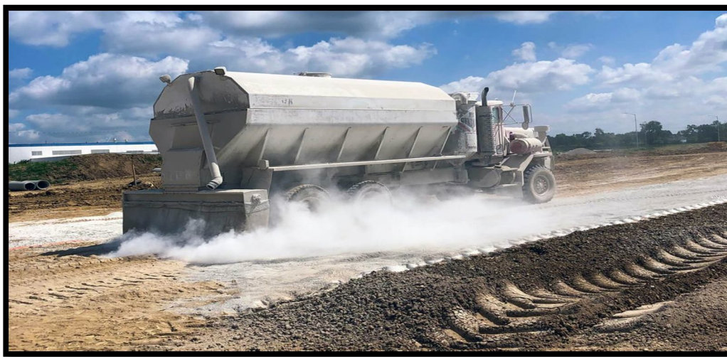
Figure. Soil Stabilization
