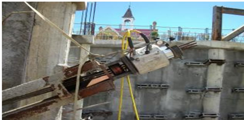
Figure 4: Testing of ground anchor
