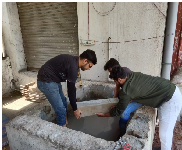
Fig. 4 Placing the blocks for curing
