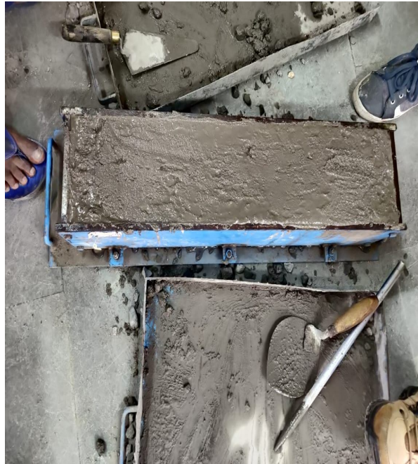
Fig. 8 Casting of concrete beam
