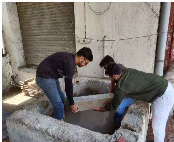
Fig. 4 Placing the blocks for curing
