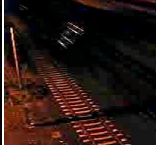
Fig. 12 Enhanced image of Railway track
