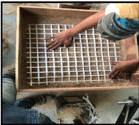
Placing of reinforcement layer
