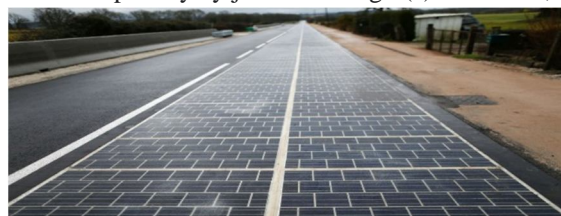
Fig 1(a) solar road
