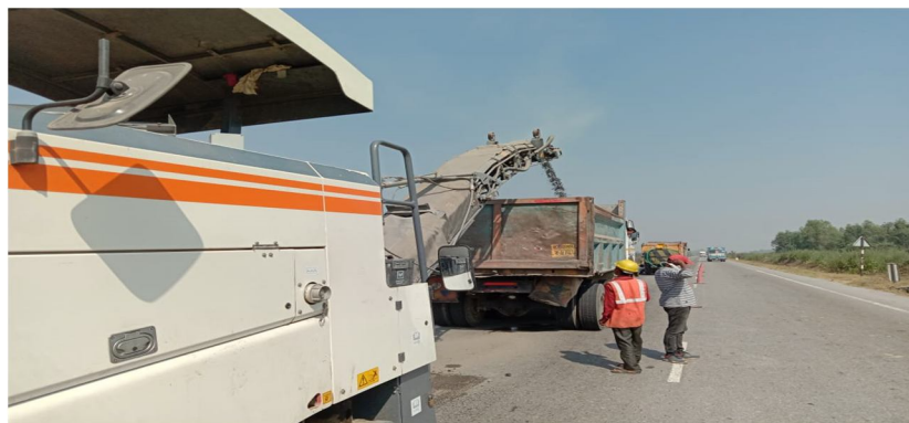
Figure 1. Cold Milling Process
