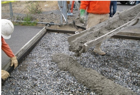
Figure 6. Recycled Aggregate Concrete For Within Site Recycling
