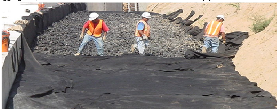
Figure 5. Recycled Aggregate as Backfill Material
