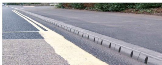
Figure 2. Recycled Aggregate as Road Kerb
