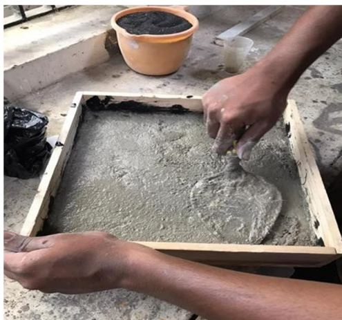
Fig.7 Finishing with Trowel
