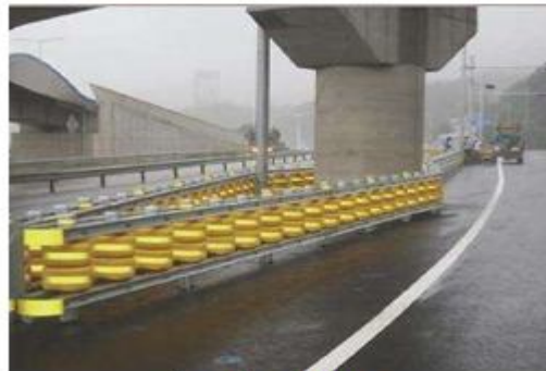
Secure a pier of a flyover
