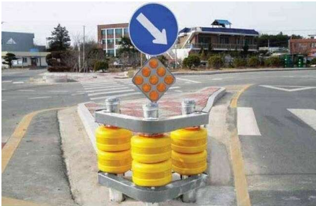
Figure.3.1.4. Rolling Barriers at the Uturn
