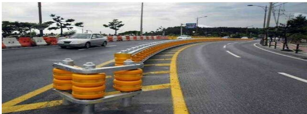
Figure.3.1.3. Rolling Barriers at the midroad and vehicle collision with diversion
