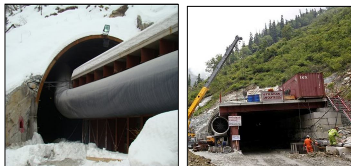
Fig 2: North and South portal of Atal Tunnel
