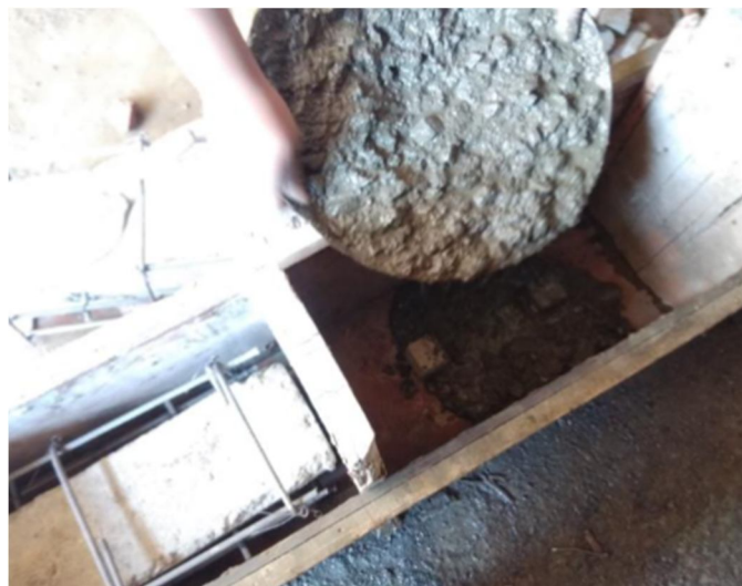
Figure 7: Filling of concrete in mould
