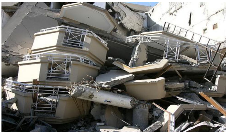
Fig. 1: A Total Collapsed Building
