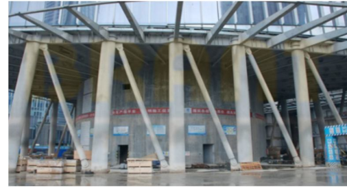
Fig.1. Buckling restrained brace
