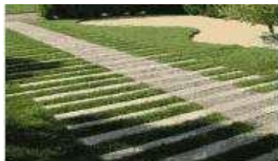
Fig. 32 A. Porous pavers to increase water percolation
