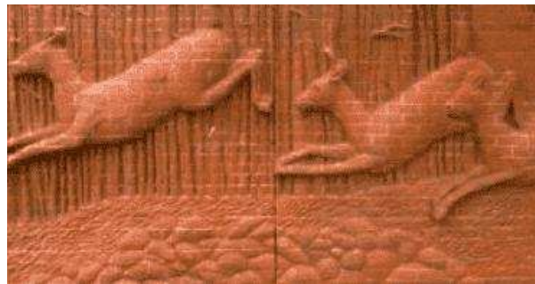
Fig. 31 C Siporex work on multilevel parking façade
