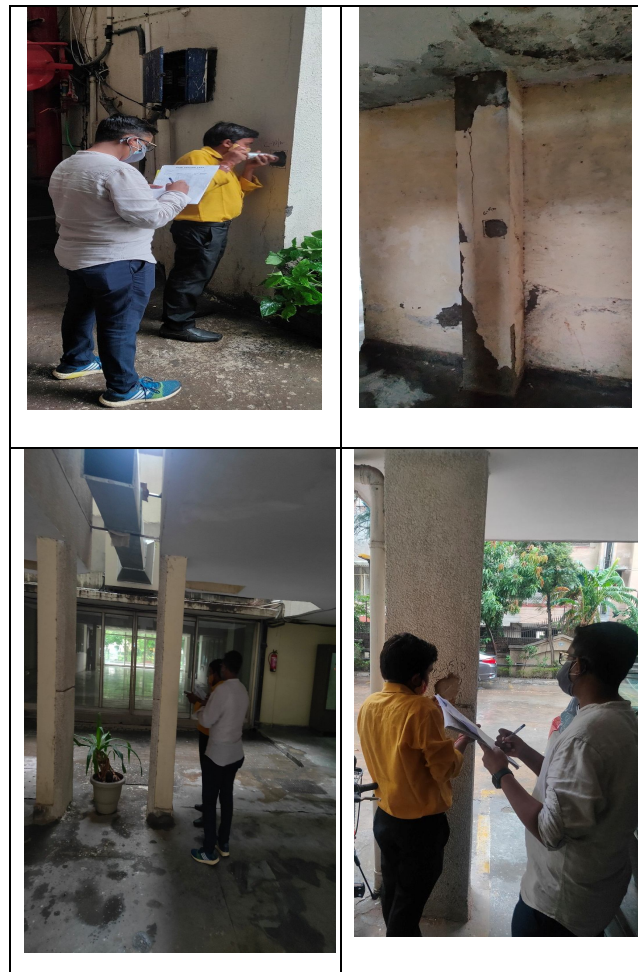
Visual Survey and Testing
