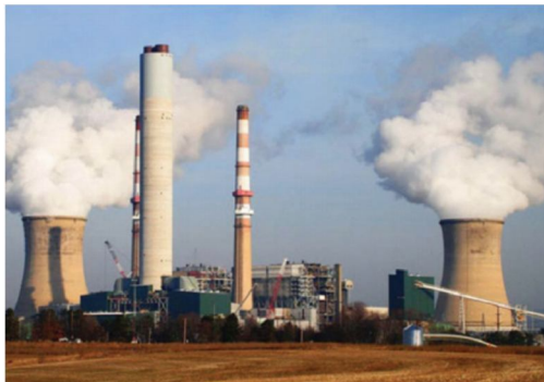
Fig. 1. Self supported steel chimneys located in industrial plant
