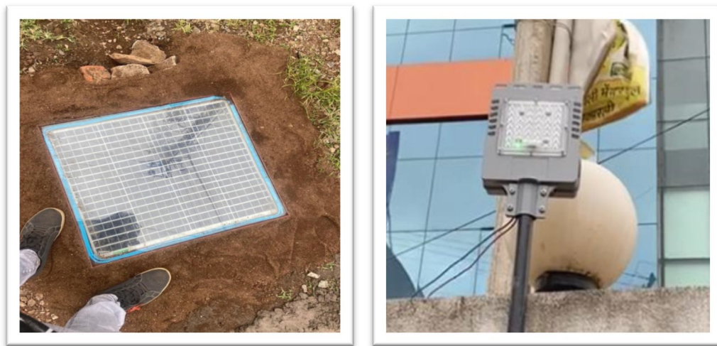
Fig.3: Installation of Solar Panel and light bulb
