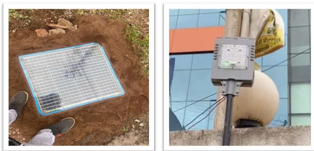
Fig.3: Installation of Solar Panel and light bulb
