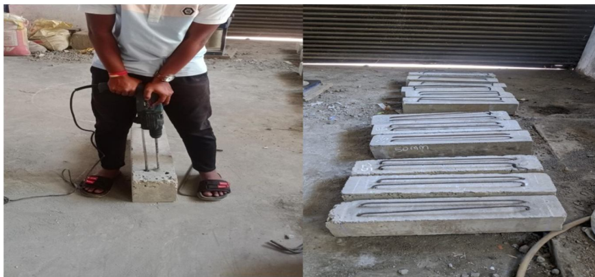
Fig No 7.2- Insertion of U shape bars in beams
