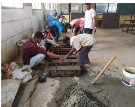
Fig No-5.1 Casting of Beam
