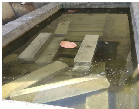
Fig No-5.2 Curing of Beam
