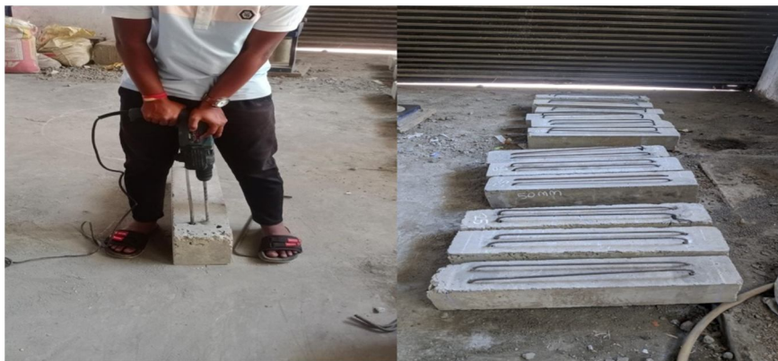
Fig No 7.2- Insertion of U shape bars in beams
