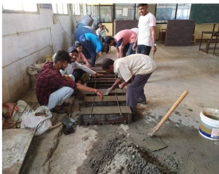
Fig No-5.1 Casting of Beam
