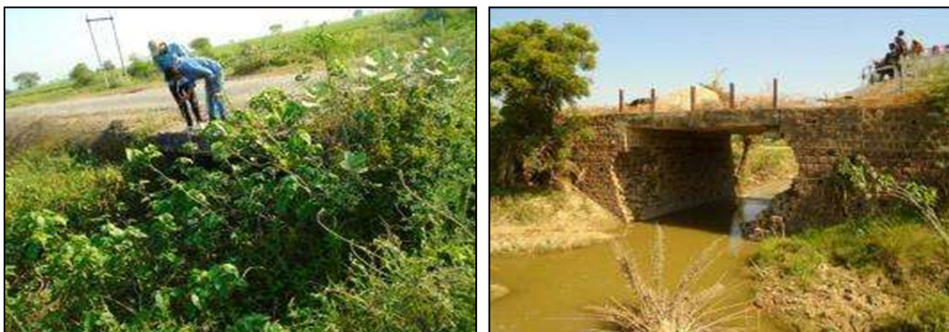
Photographs showing existing Slab culverts on the Project Road
