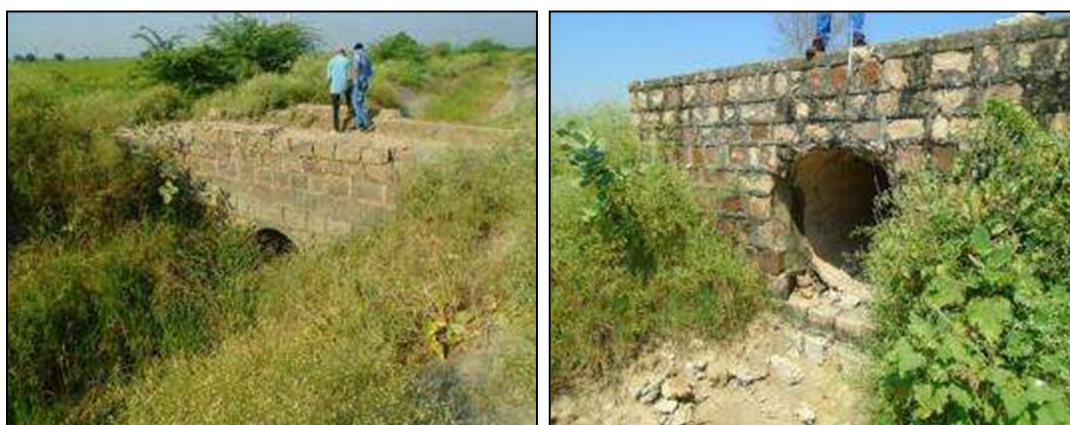
Photographs Showing Pipe Culverts on the Project Road
