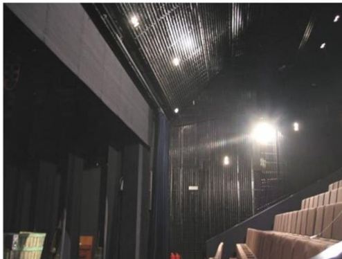
Fig 7 The interior of Room 4
