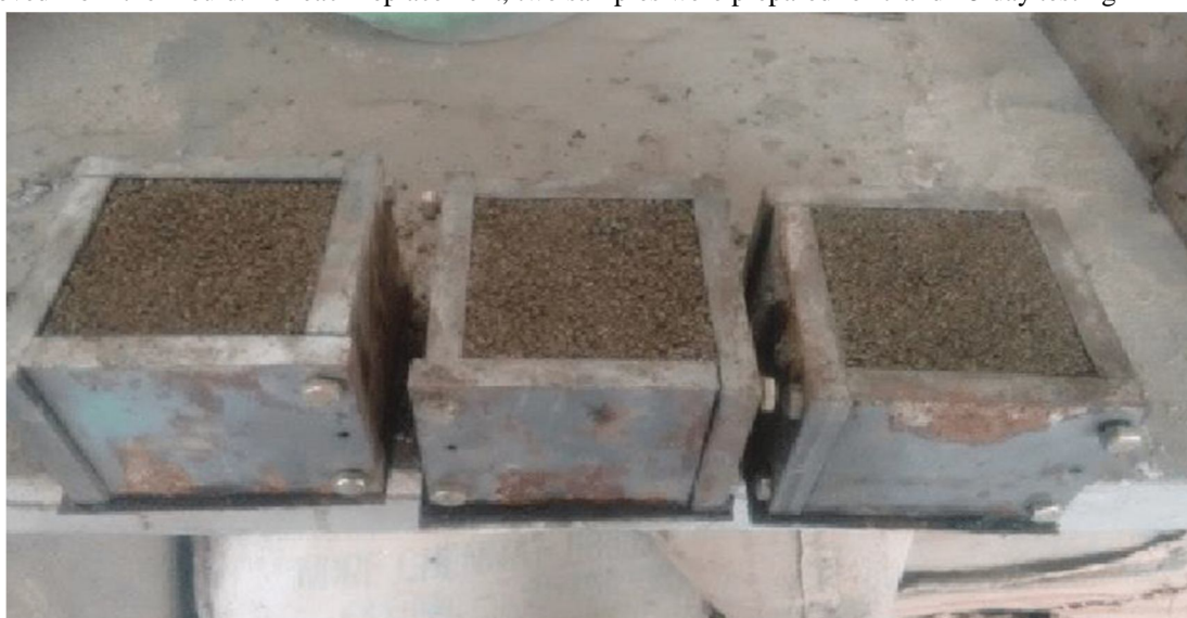
Fig showing compaction and surface finishing of the cube
