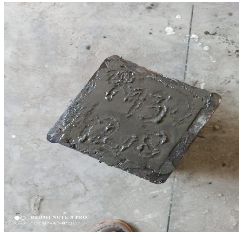
Figure 1: Casting of concrete cubes
