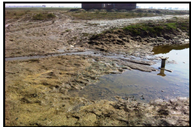
Photo No.6. Photograph showing water logging control by lane pattern at Baghpur village
