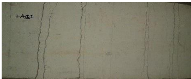
Figure 5.2 evenly distributed crack pattern in FCCG
