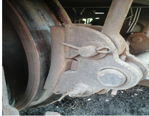
Fig 2: CONDITION OF BRAKE SHOE
