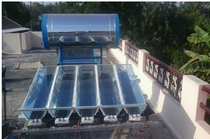
Fig no: 3 Construction of v-trough
