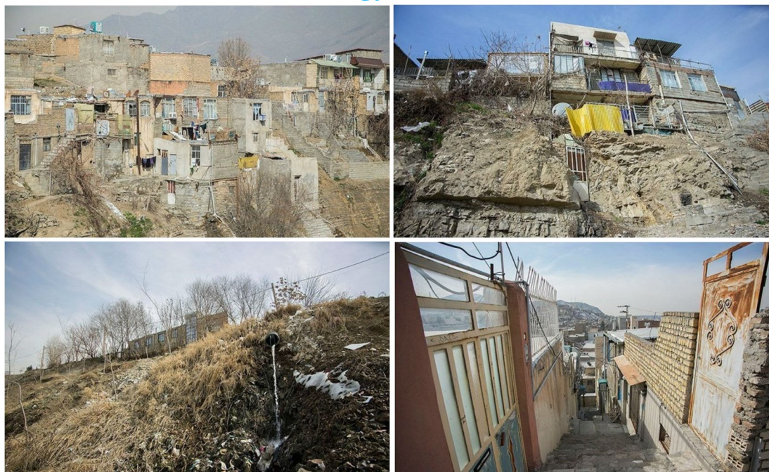
Figure 4: structure and environmental qualities of Hesar neighborhood (Source: Tasnim agency: http://www.tasnimnews.com/fa/media )
